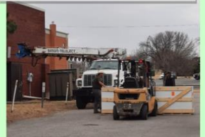
Air conditioning parts arrived!
